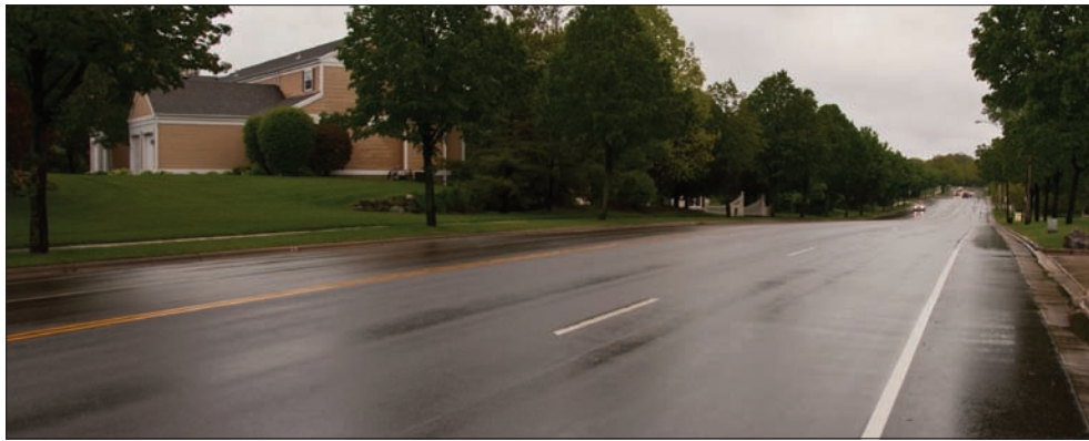
Collaboration to Enhance Wisconsin's Local Roads
